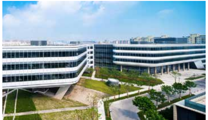
Johnson Controls Headquarters Asia Pacific in Shanghai, China.
