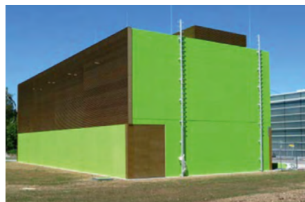
New technical building with transformer station, four cooling towers and building automation facility.
